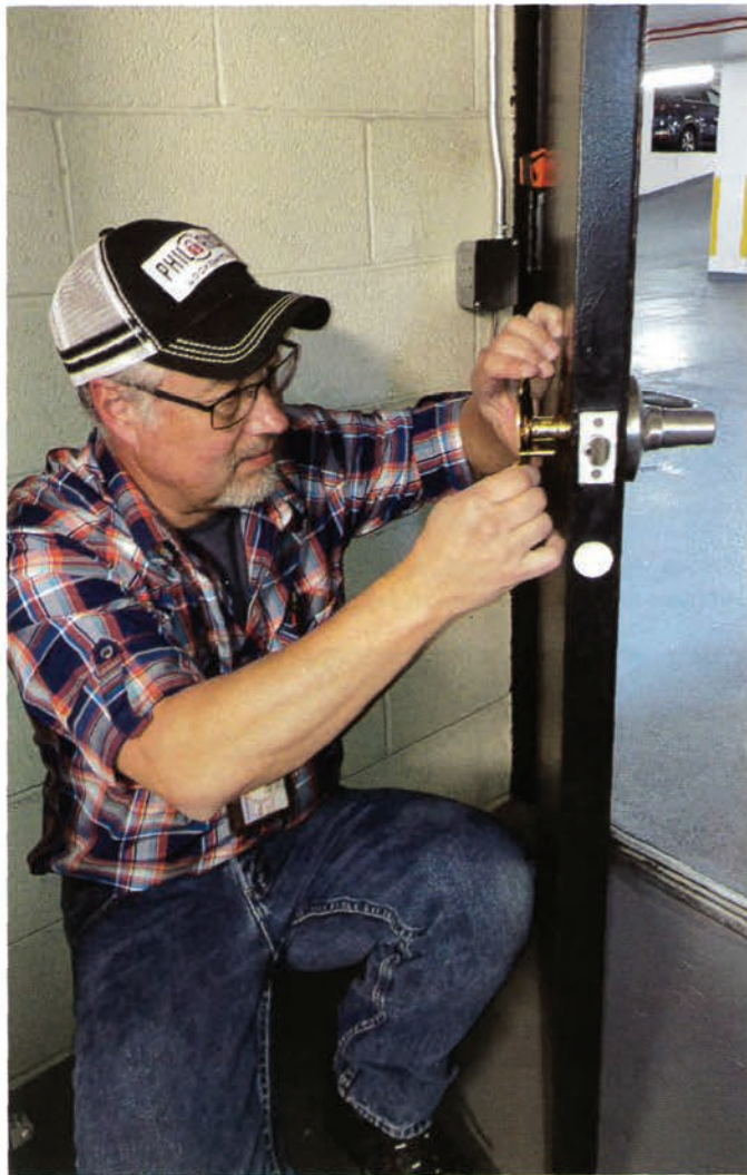
Figure 23. The author is installing the lock.
