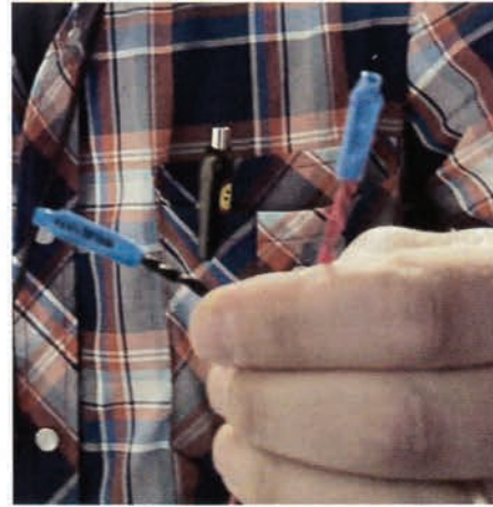
Figure 22. The author is connecting the red and black wires from the lock to the power wires in the door.
