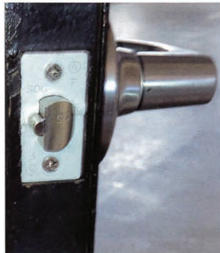
Figure 20. The latch is installed.
