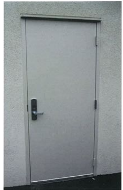
Exterior side of door
