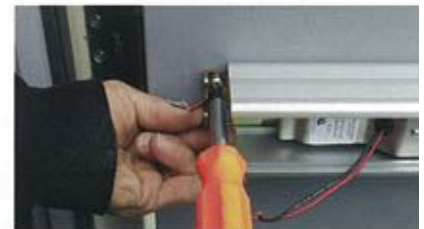
Install mounting bracket
