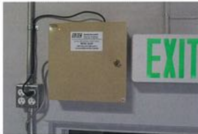
Power supply installed above door
