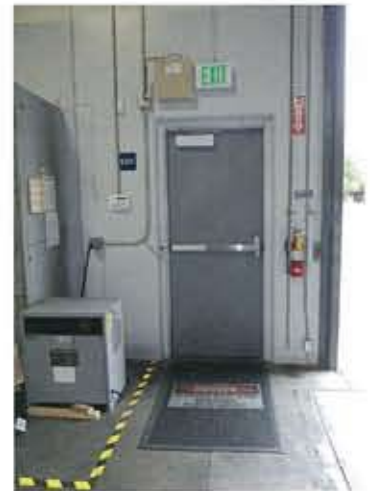
Finished installation, interior
