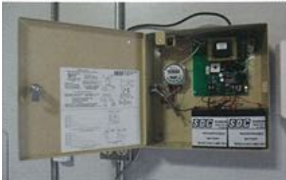
Install power supplier, timer & batteries
